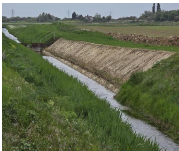
Completed Revetment works April 2025
