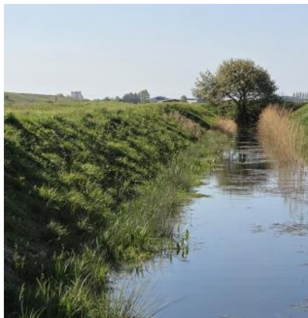
Re-established Revetment works, reach 6a – 7 April 2026
