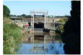
• Old Bedford Sluice
