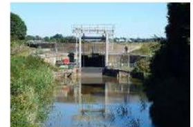
• Old Bedford Sluice
