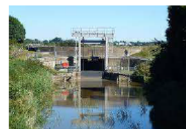
• Old Bedford Sluice
