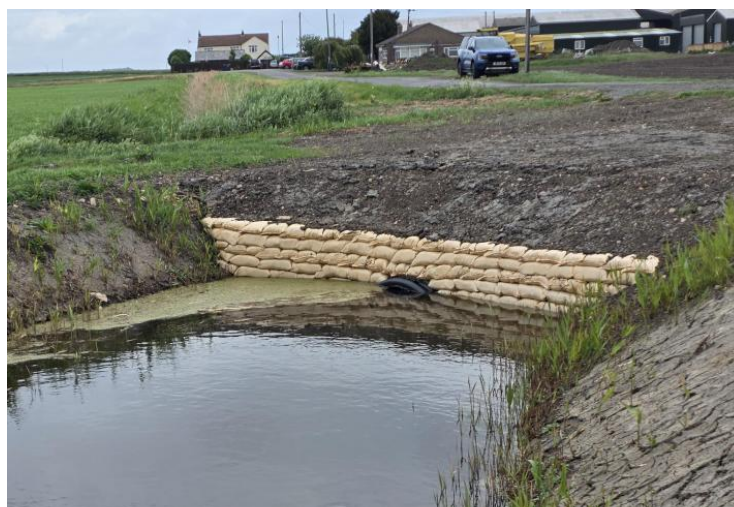
Fully funded, replacement culvert at Point 11
