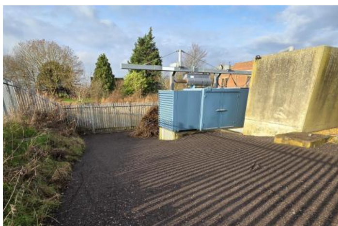
Fully funded improvement works at Pumping Station
