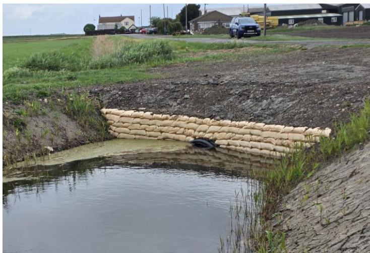
Fully funded, replacement culvert at Point 11
