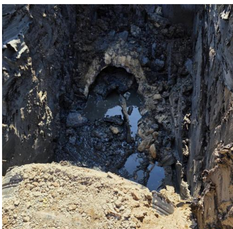
Point 52, Culvert Replacement. New 1800mm pipe in the bottom of picture & old silted up 900mm pipe in the top.
