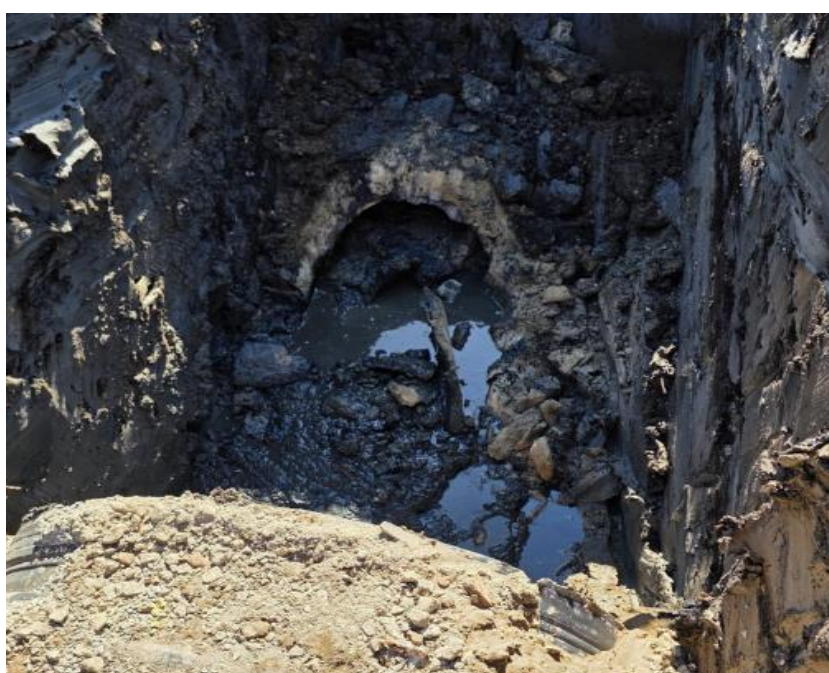
Point 52, Culvert Replacement. New 1800mm pipe in the bottom of picture & old silted up 900mm pipe in the top.
