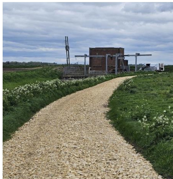
Improved access road to Pumping Station
