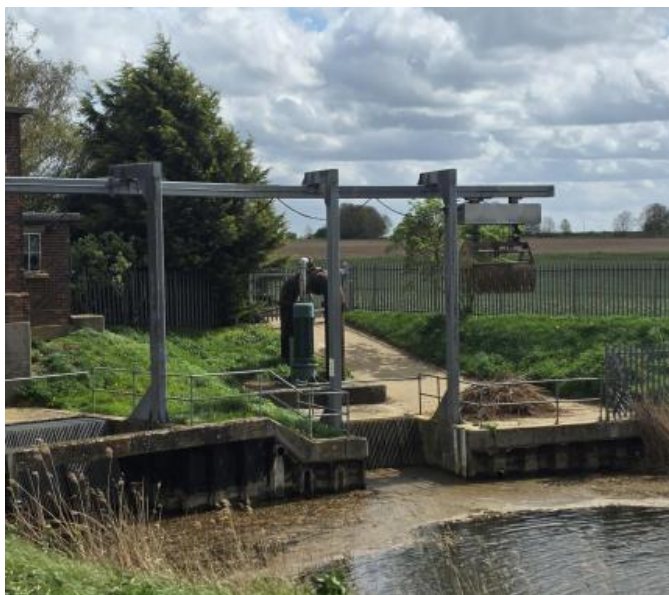
Improvements works @ Latches Fen Pumping Station
