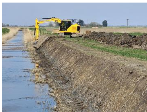
Bank revetment works in progress, reach 52-53
