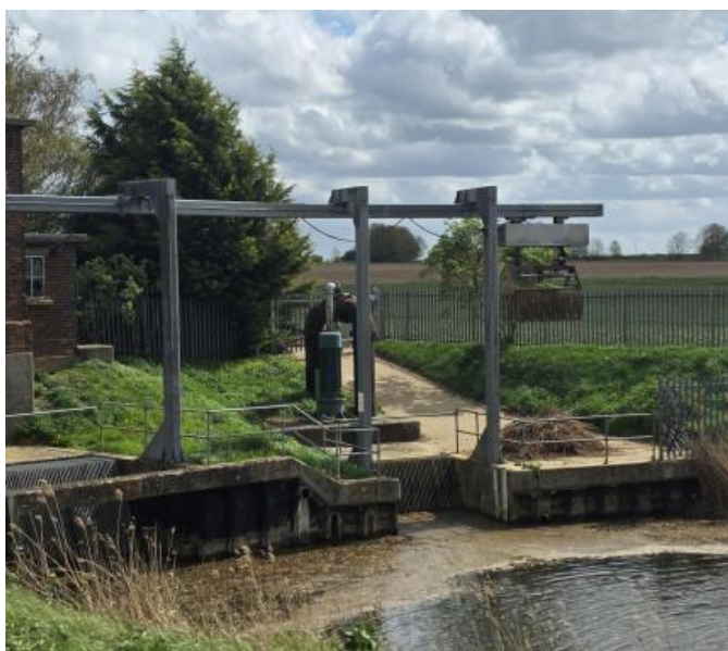
Improvements works @ Latches Fen Pumping Station
