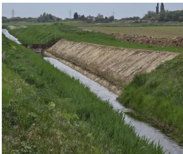
Completed Revetment works April 2025
