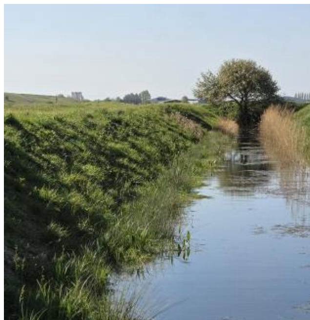
Re-established Revetment works, reach 6a – 7 April 2026
