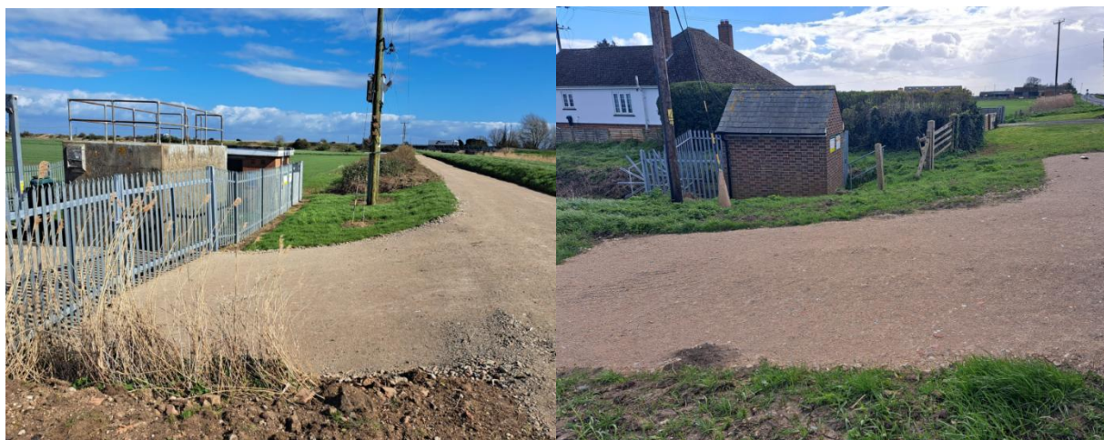
Curf & Finchams Pumping Station improvements works above.
