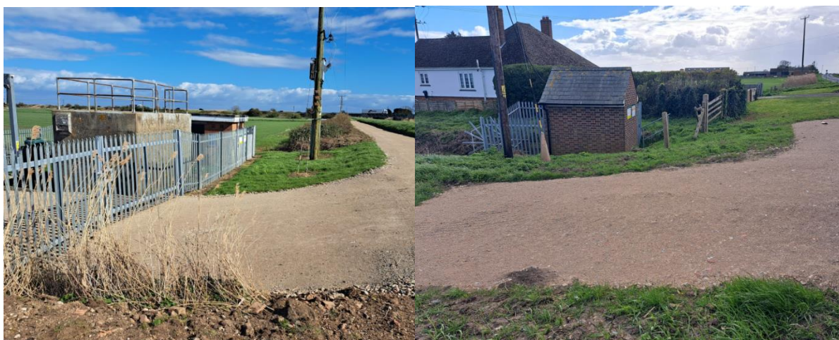
Curf & Finchams Pumping Station improvements works above.
