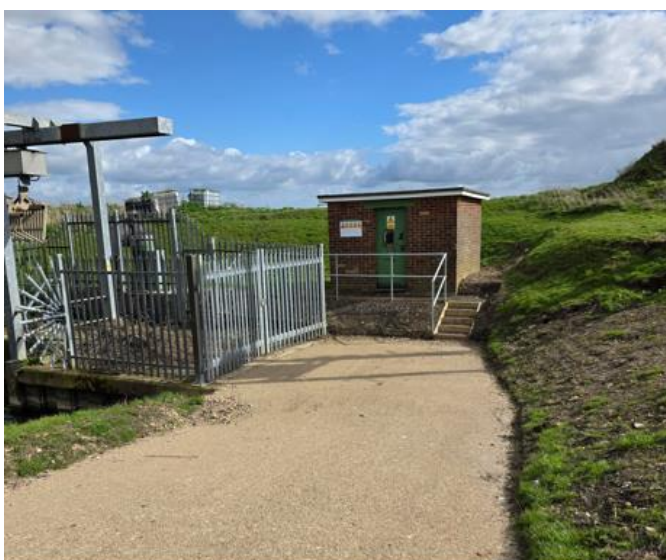
Health & Safety remedial works and access improvements at West Fen Pumping Station for deployment of Mobile Pumps in the event of a breakdown
