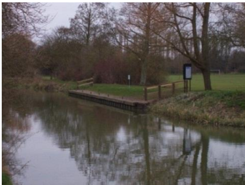
Adjacent Manor Leisure Centre, Whittlesey – Kings Dyke
