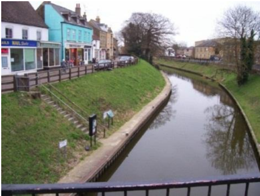
March Town Centre Bridge – Old River Nene Mooring
