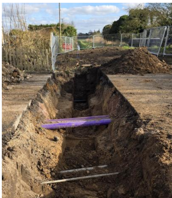
Point 50, road crossing & numerous services exposed during works
