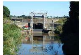
• Old Bedford Sluice
