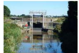
• Old Bedford Sluice
