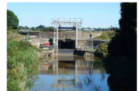
• Old Bedford Sluice
