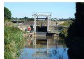
• Old Bedford Sluice
