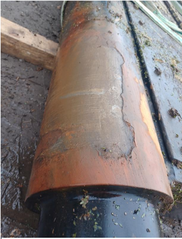
Photo showing damaged door post at Marmont Priory
