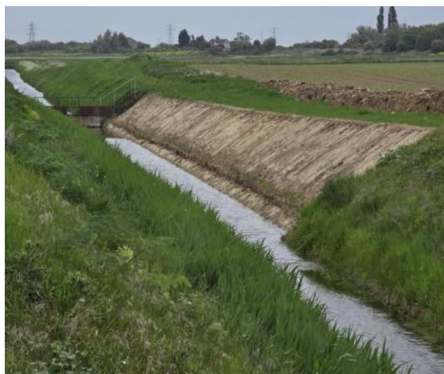
Bank Revetment works & coir roll installation, reach 6a-7
