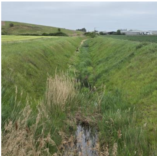
Natural reed bed, EEDA drain reach 19-20
