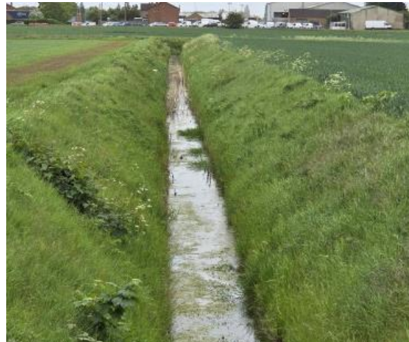
Emergent aquatic vegetation due to be machine cleansed this season, reach 14-15
