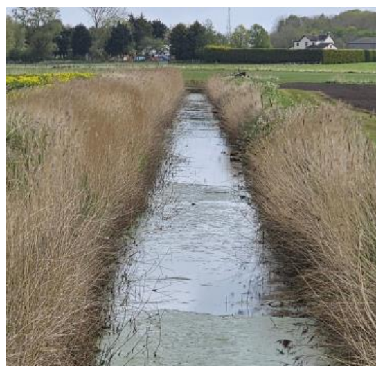
Well maintained drain, with good marginal vegetation
