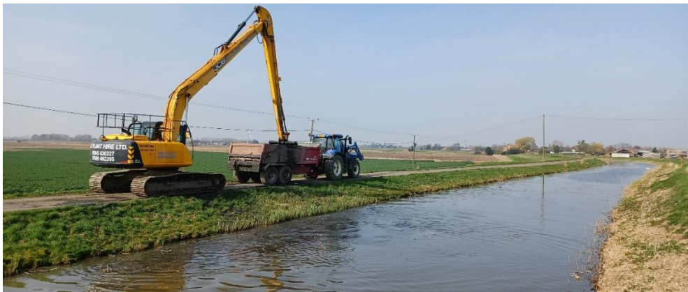
Well Creek Phase VII Dredging Works – Nordelph Village to Mullicourt Aqueduct
