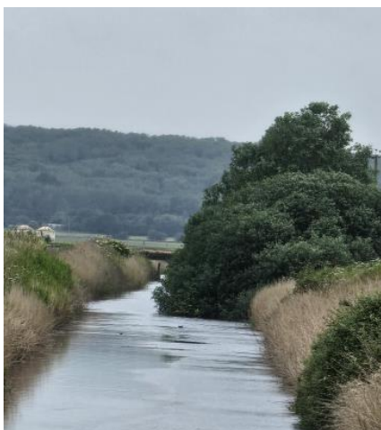
Ash Drain Saplings, reach 8-9
