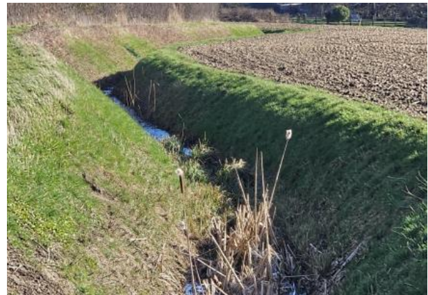
Reach 42-43, to be monitored for maintenance requirements
