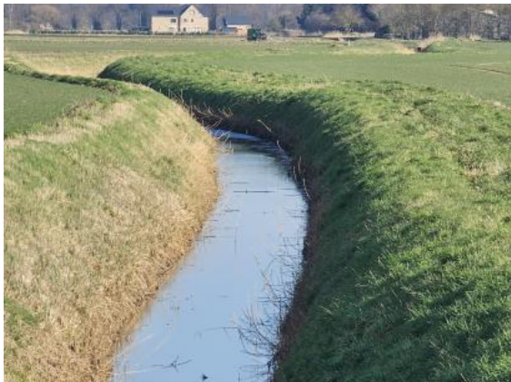
Clear drains along Reach 40-41
