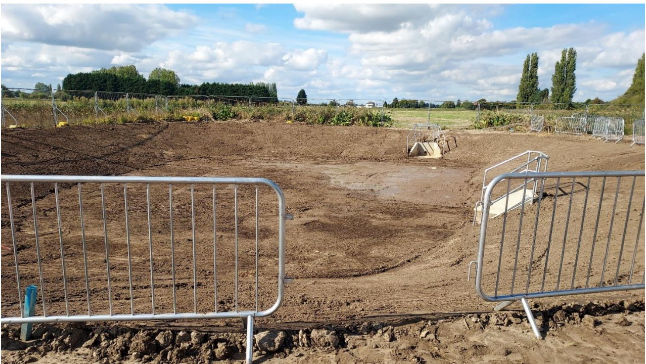
A view of the empty attenuation basin
