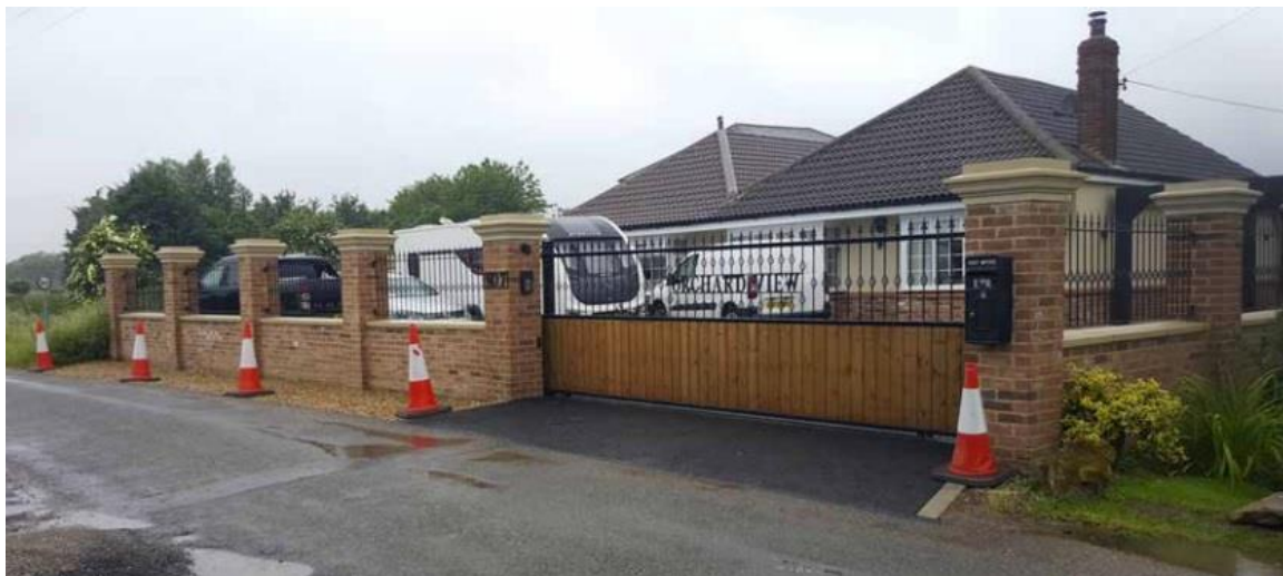
Photograph of the site included within Acstro Limiteds Access Appraisal.
