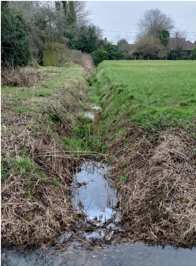
Recent view of the new cut channel
