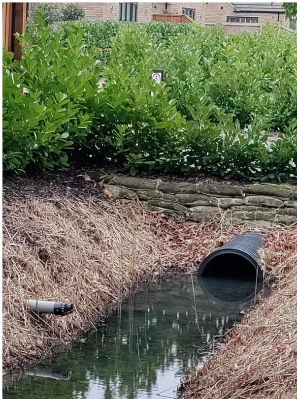
An outfall from one of the new dwellings
