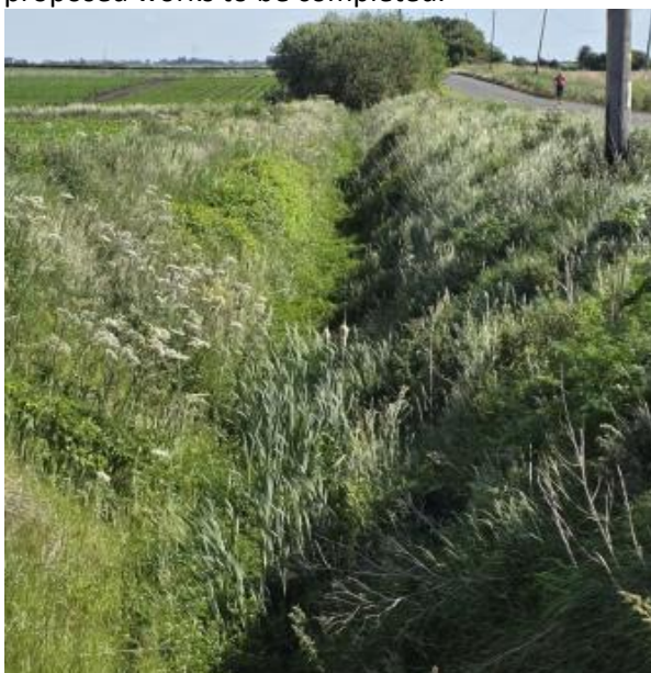
Hollow Head spur drain, reach 73-74
