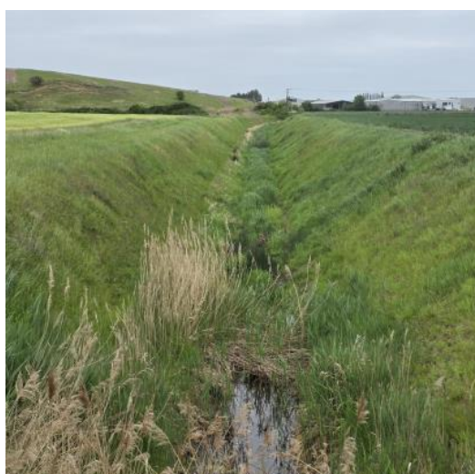
Natural reed bed, EEDA drain reach 19-20
