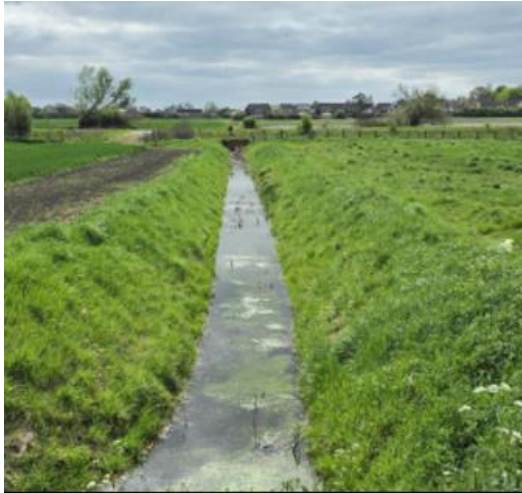
Aquatic vegetation evident in reach 29-30
