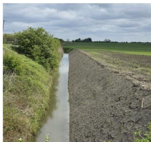
Revetment works, Reach 18-19
