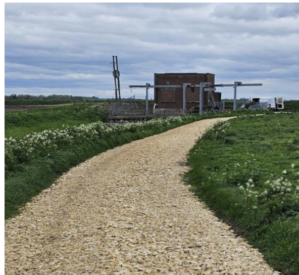
Improved access road to Pumping Station
