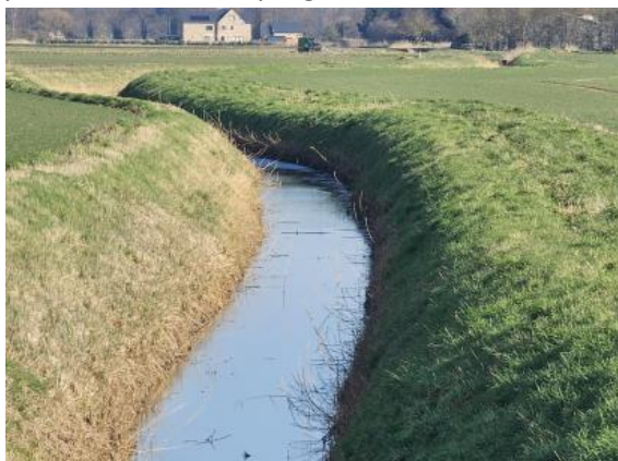
Clear drains along Reach 40-41
