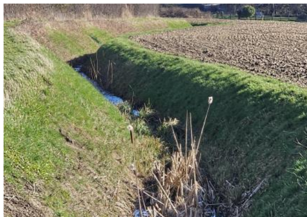
Reach 42-43, to be monitored for maintenance requirements
