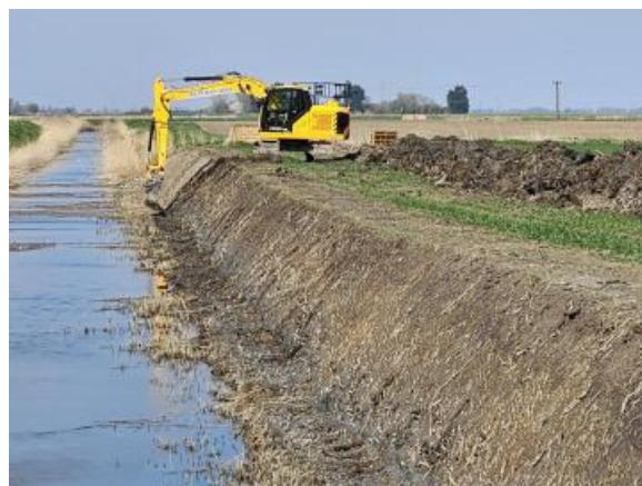
Bank revetment works in progress, reach 52-53
