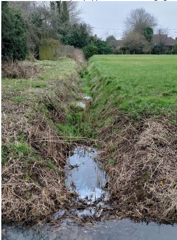
Recent view of the new cut channel
