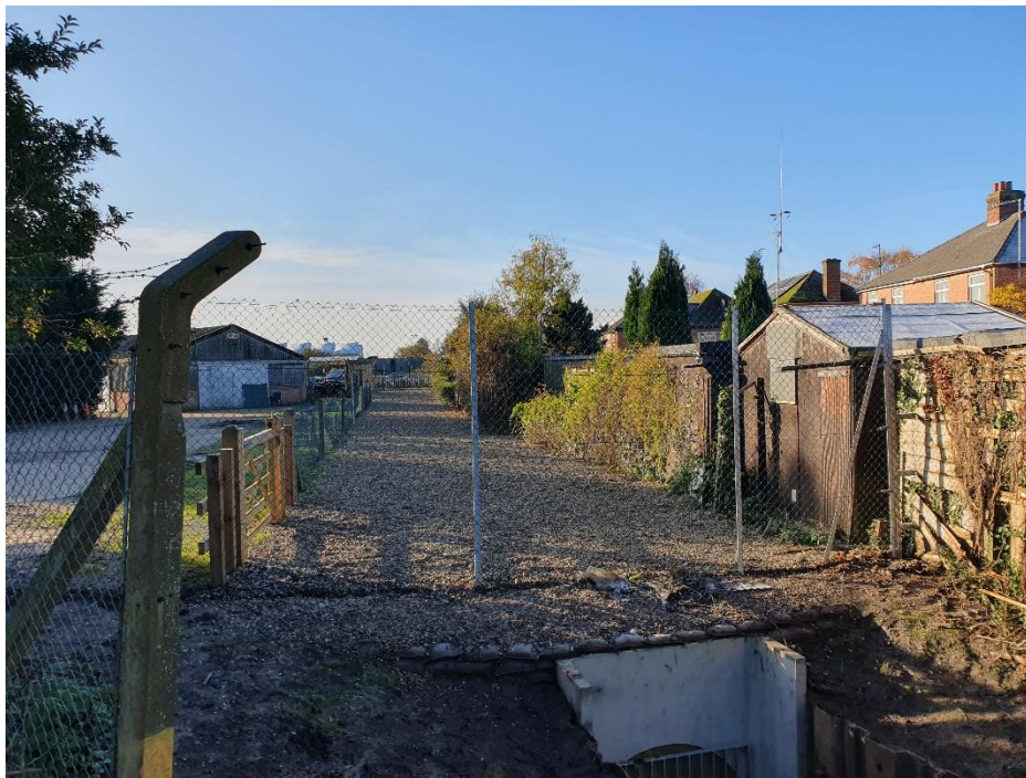
Completed works looking downstream, from the upstream extent
