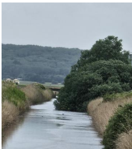
Ash Drain Saplings, reach 8-9
