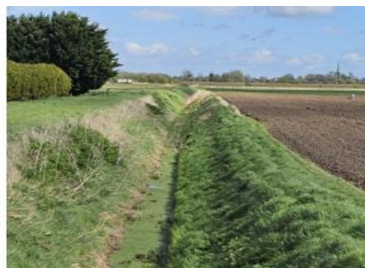
Cross Road, reach 14-15
