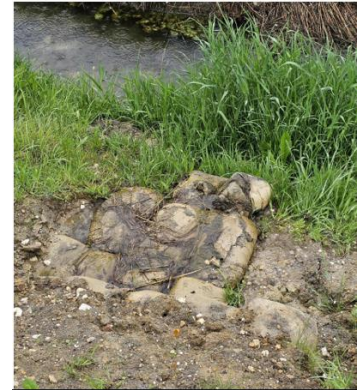
Discharge spillway, Point 20
