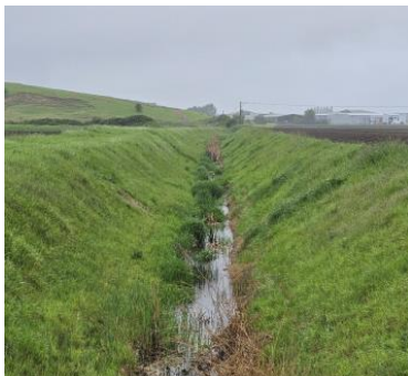
Emergent aquatic vegetation, creating a natural filtration system, reach 19-20
