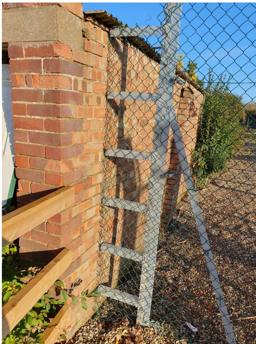
Improved chain link fencing at downstream end
