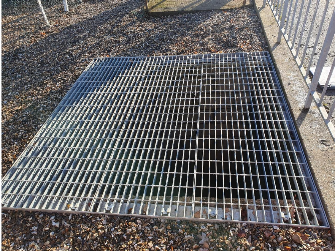
Corrected inspection chamber grills and brackets with security bolts
