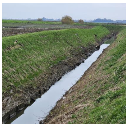
Deteriorating revetment,
