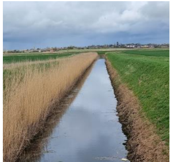
Typical example of the alternate sides @ Point 81
