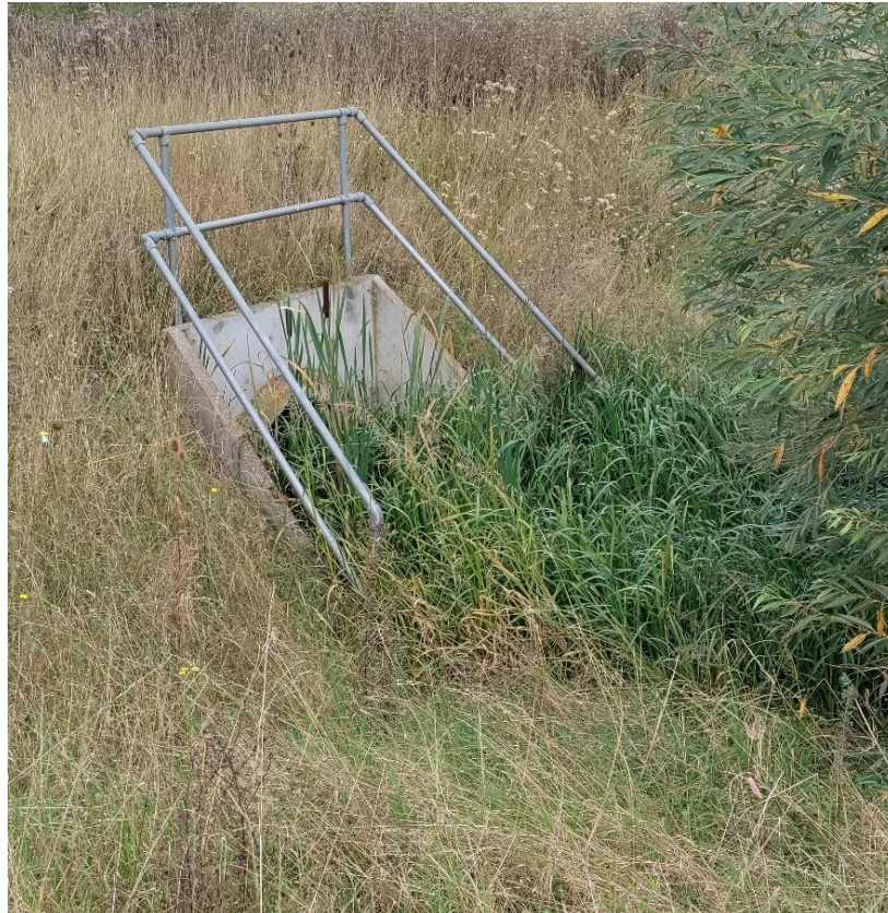
Upstream end of the surface water outfall
