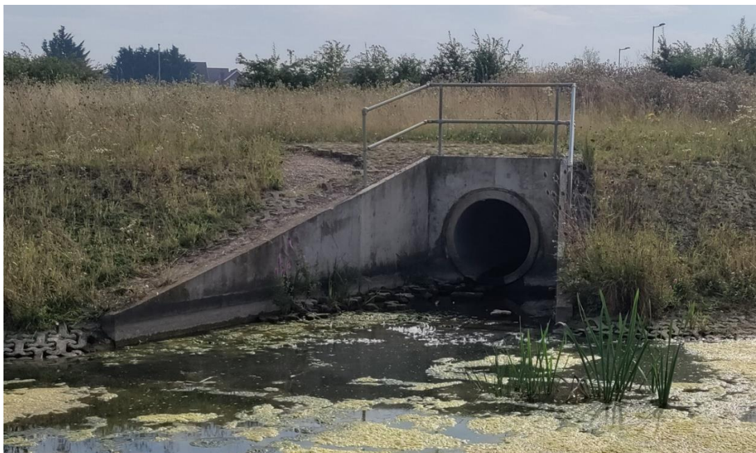
The surface water outfall viewed from the western side of the channel
