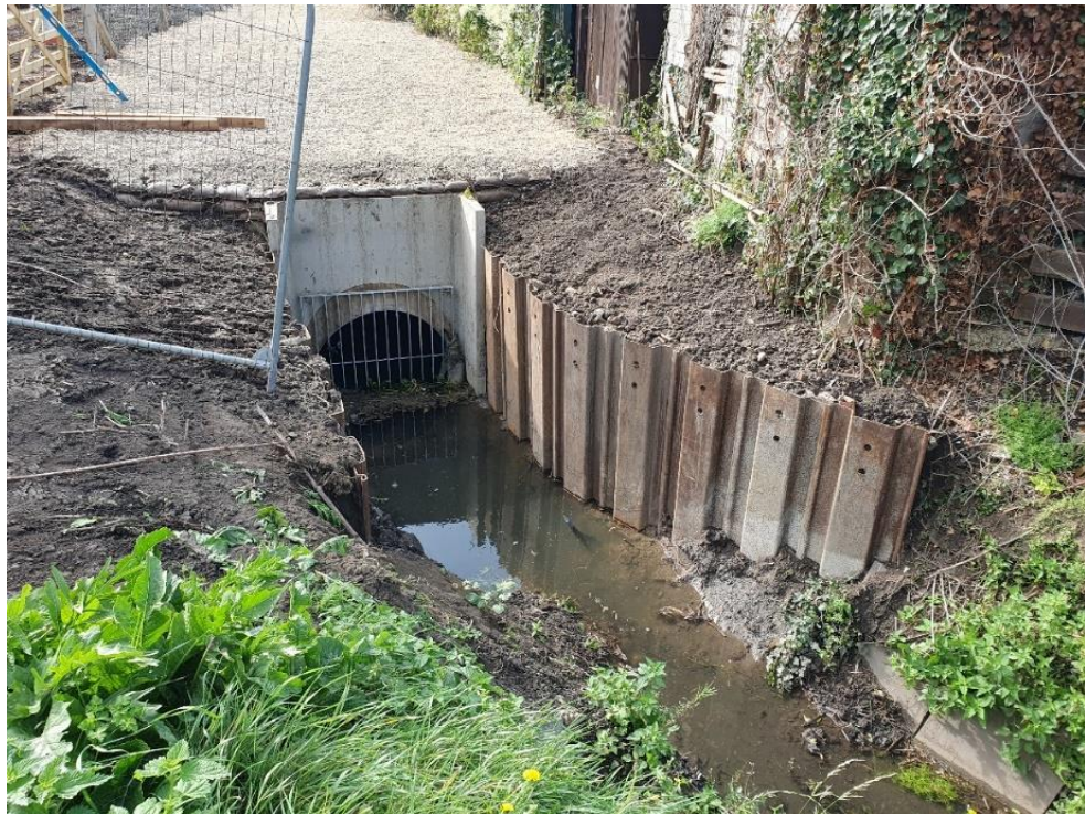
Headwall and piling at upstream end
