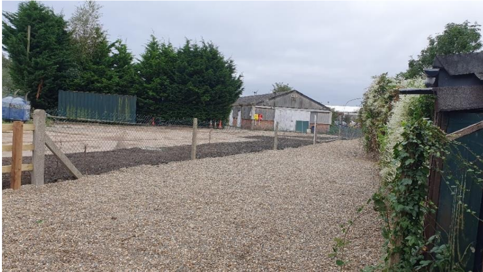
Area culverted looking downstream, from the upstream extent
