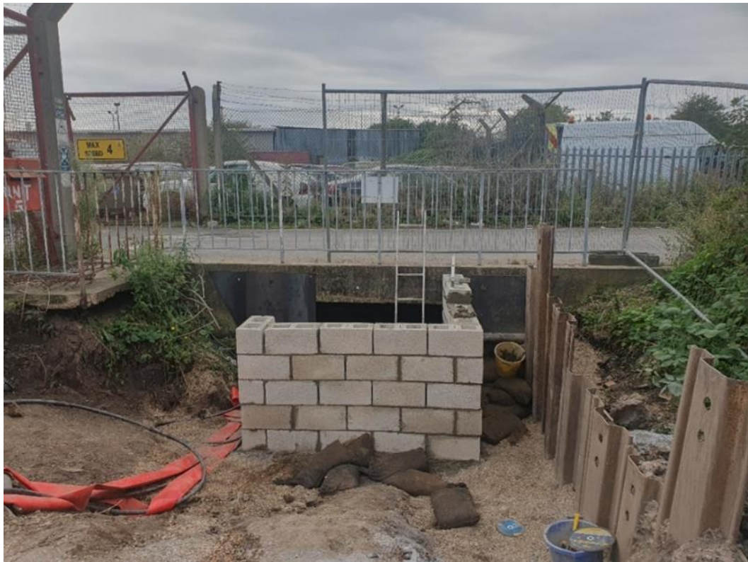
Chamber at downstream end during construction and adjacent piling for additional garage support
