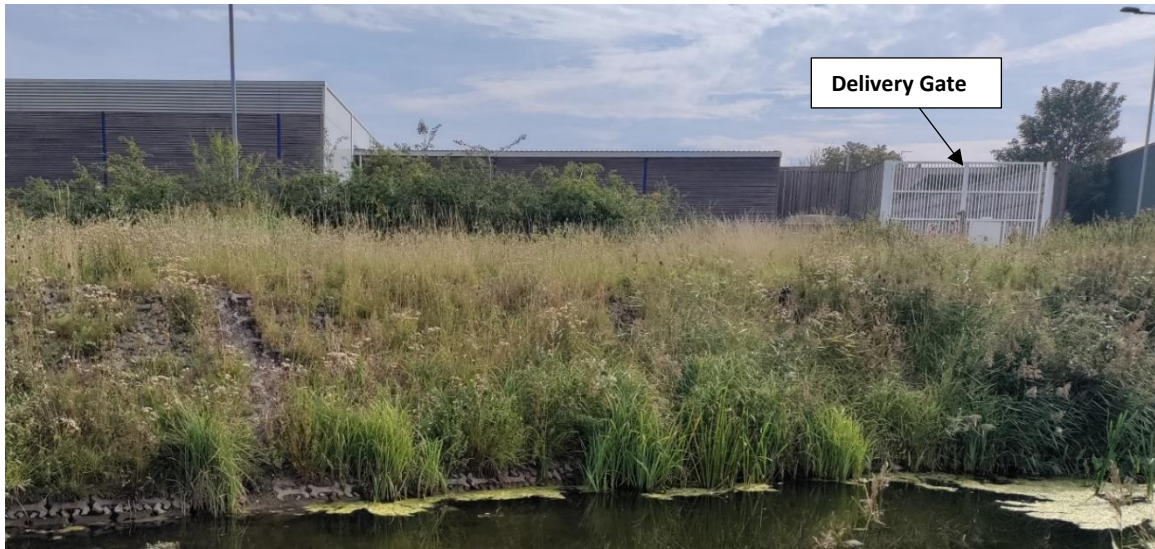
View of the steep hard revetment
