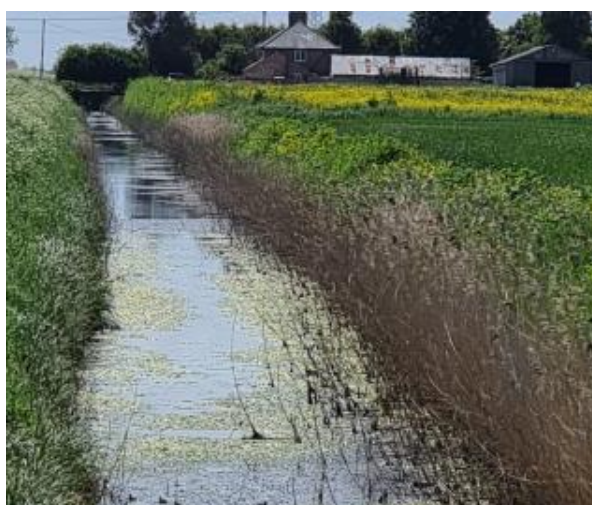
Long Drove Drain, reach 12-13
