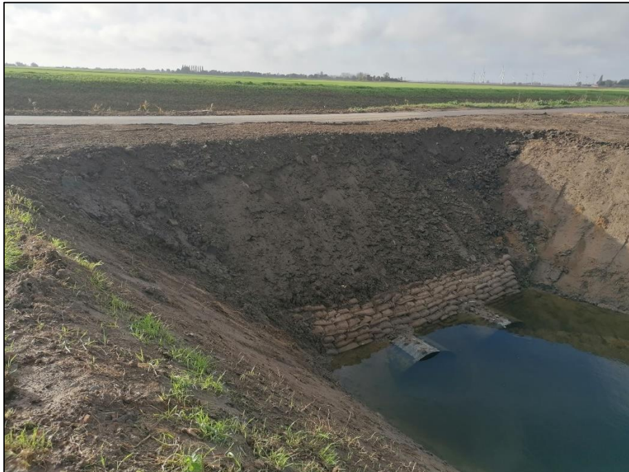
Completed Main Outfall Culverts Installation at Point 1 on Upstream Side
