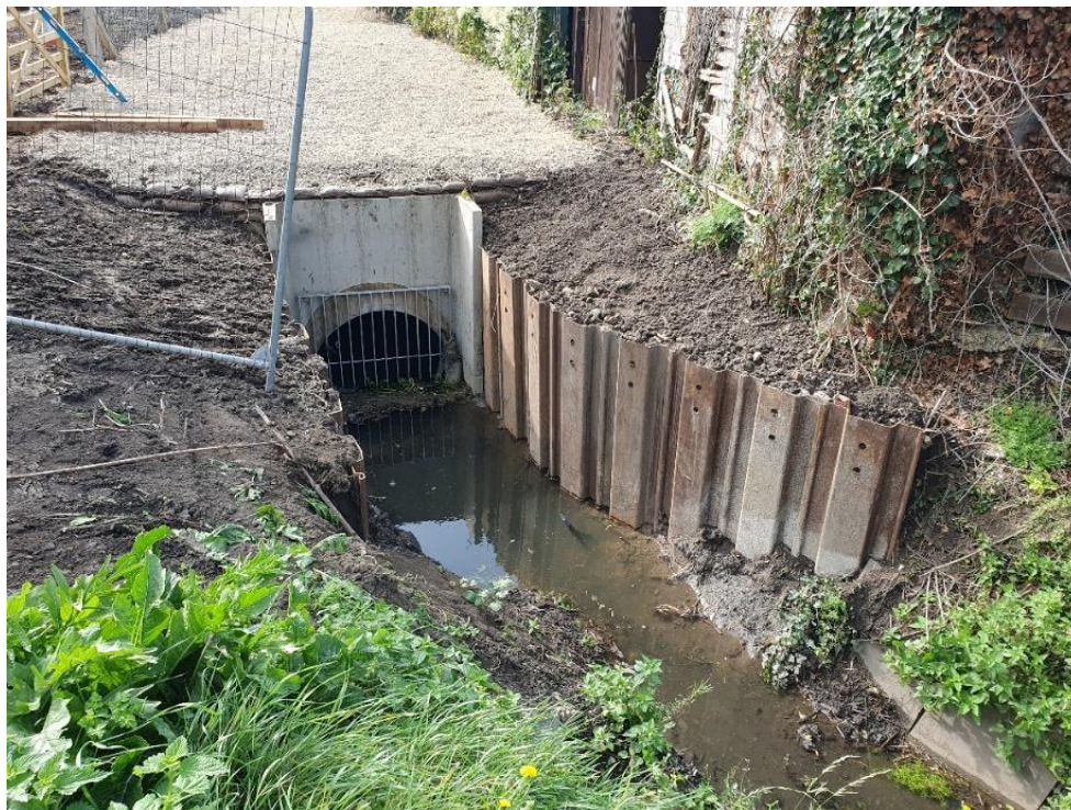
Headwall and piling at upstream end
