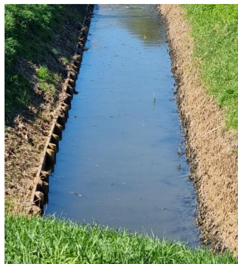
Revetment works, Point 38
