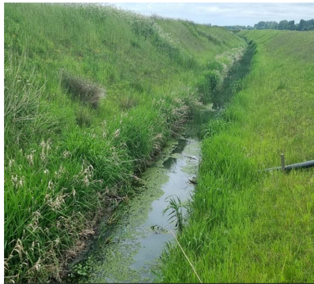
Downstream of Culvert discharge, reach 19-20
