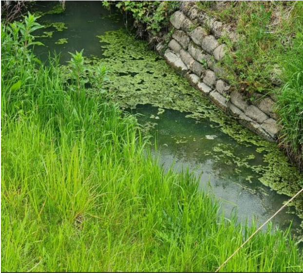
Point 20 Culvert discharge
