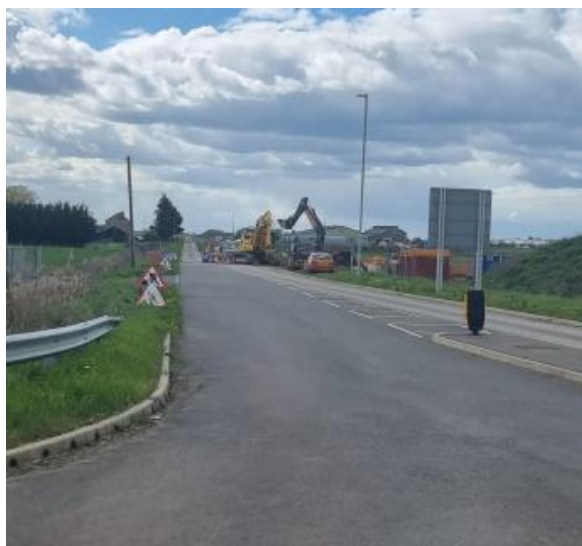
Lagoon connection under Gaul Road, Reach 10-21
