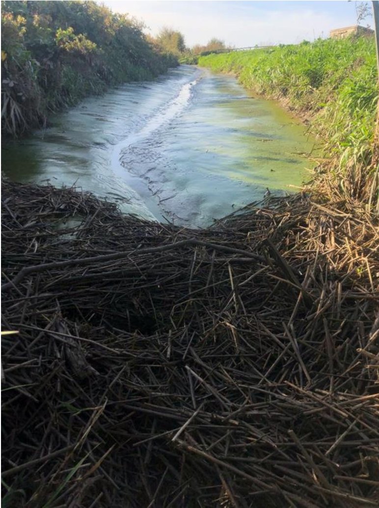
Fig 2: Header Drain from Hagen Smarts slacker, prior to slubbing out.
