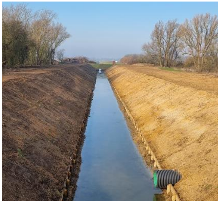
Wimblington Common Pump Drain revetment works, reach 41-42
